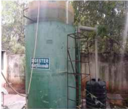
Bio Gas generation
