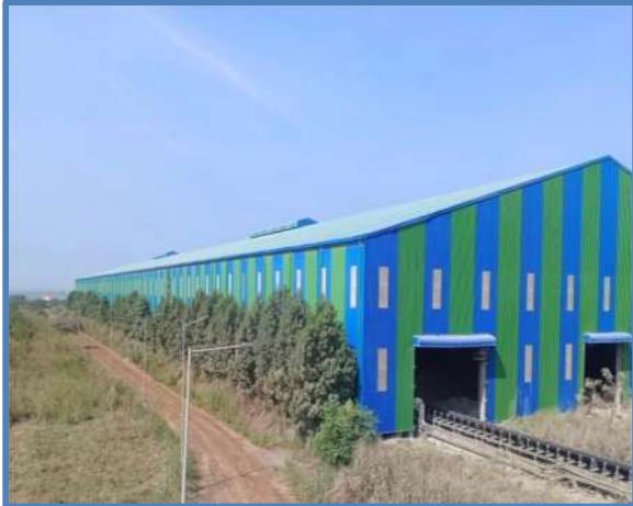
Closed Limestone Storage Shed
