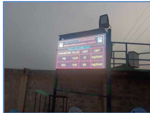
Displaying of Stack emission
