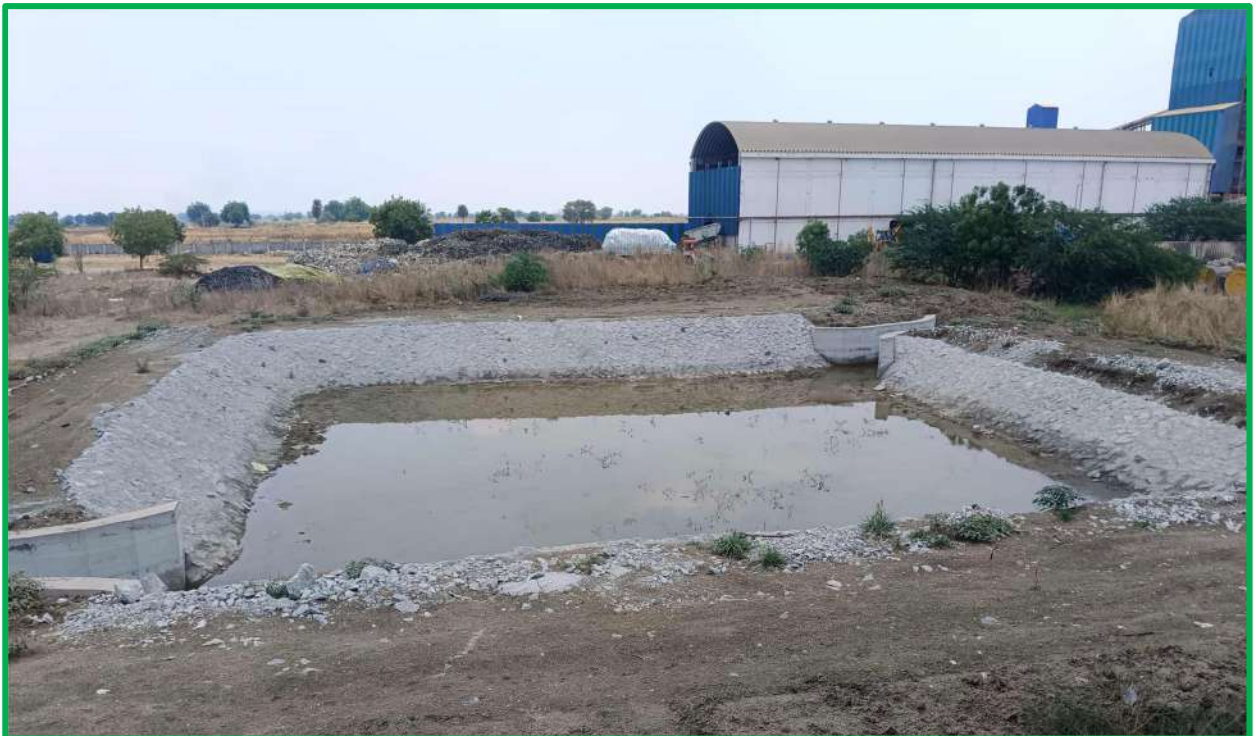
Rain water harvesting structure developed in plant area
