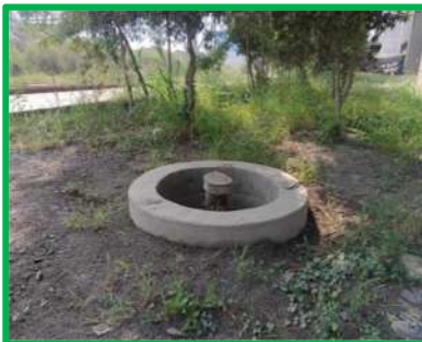
Clinker Silo Area
