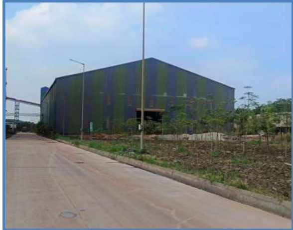
Closed Additive Storage Shed
