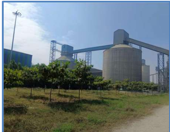
Silo for Clinker Storage – 2 X 50,000 MT
