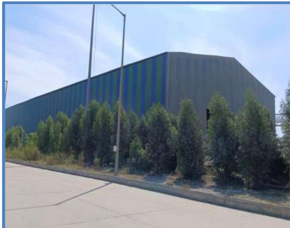
Gypsum storage shed
