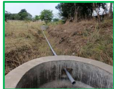
Admin Building Area
