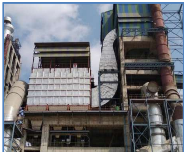
Bag House for Cement Mill
