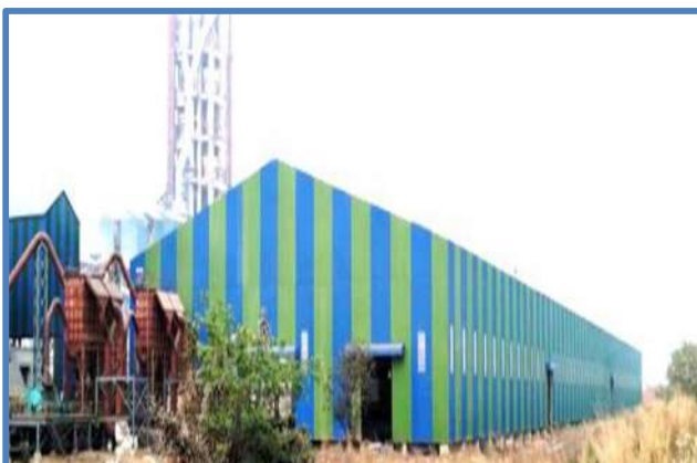
Coal Storage Shed Construction Completed
