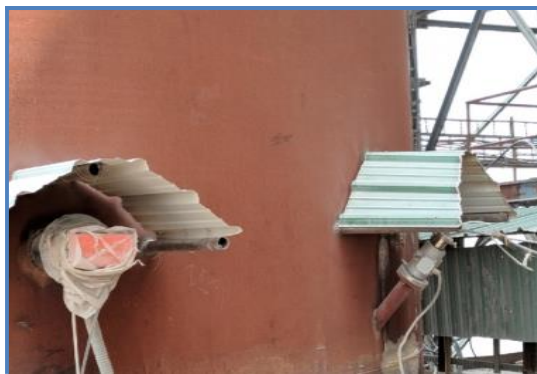
PM & Gaseous CEMS for Kiln & Raw Mill RABH Stack
