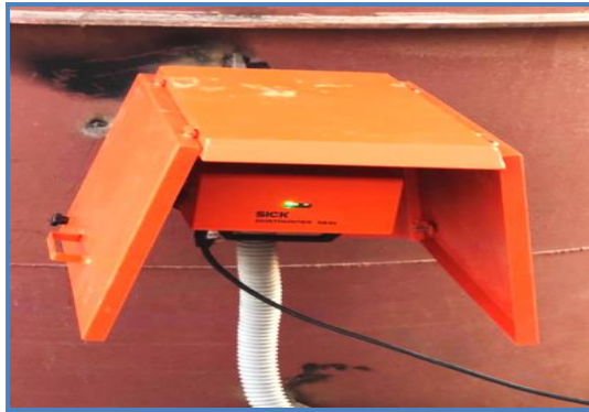
PM CEMS for Coal Mill Bag House Stack
