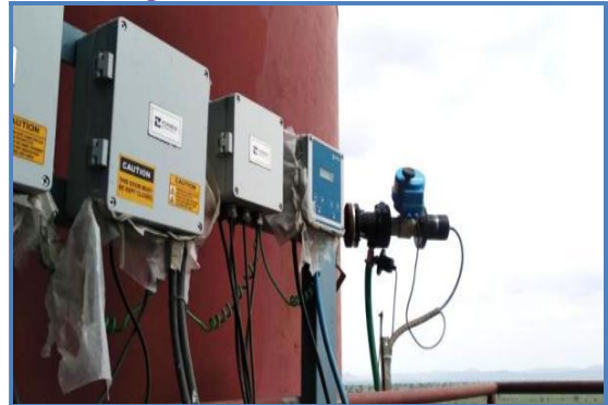
PM CEMS for Cement Mill Bag House Stack
