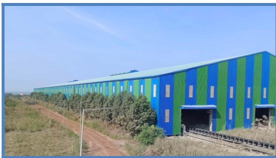
Closed Limestone Storage Shed
