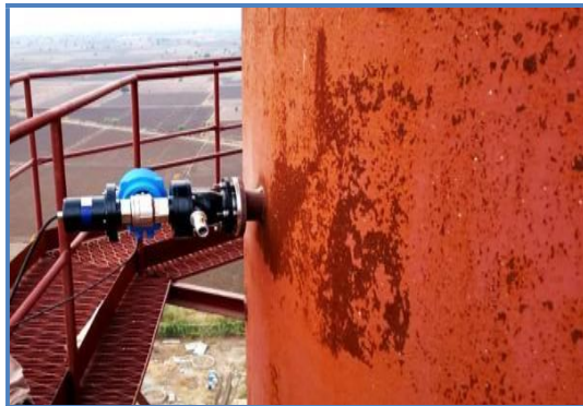
PM CEMS for Clinker Cooler ESP Stack
