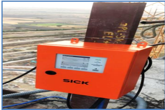
PM CEMS for Coal Mill Bag House Stack
