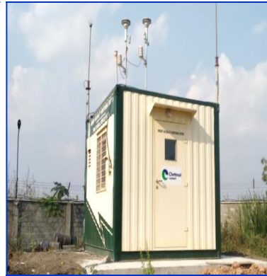
CAAQM-2 @ Project Office
