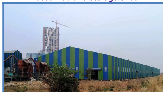
Coal Storage Shed
